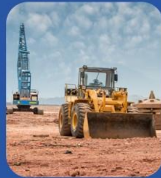
NO.3 Construction site
