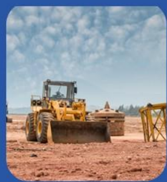
NO.3 Construction site
