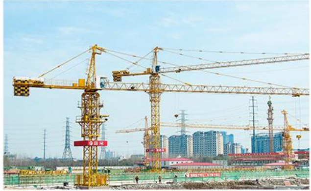
Tower crane site
