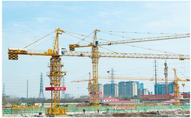
Tower crane site
